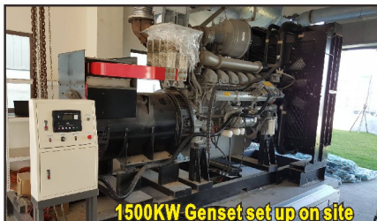
1500KW Genset set up on site
