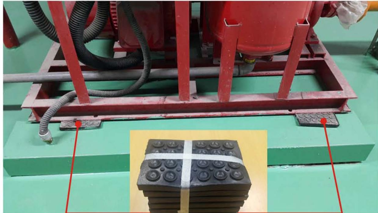
**Put 4 Shockproof Pads on the 4 corners of Fire-fighting pump sets.**
