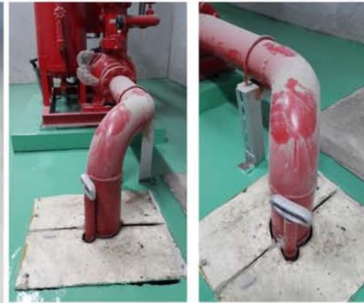
**Installed Main Piping on Pump Suction**
