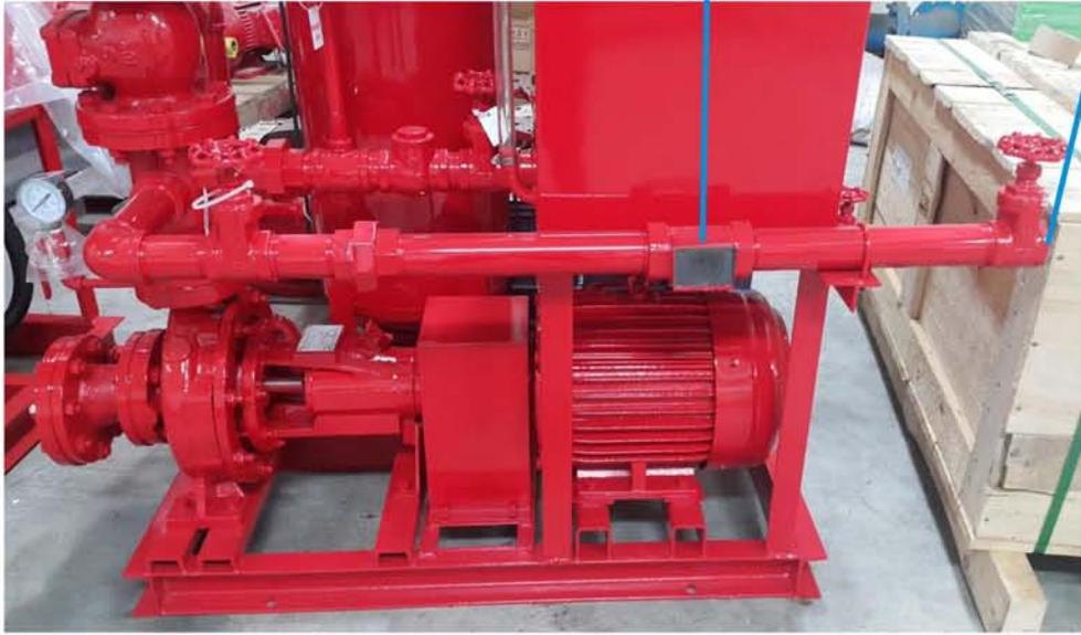
**Installed discharge pipe on Flow Meter pipeline, to drain water when testing flow**
