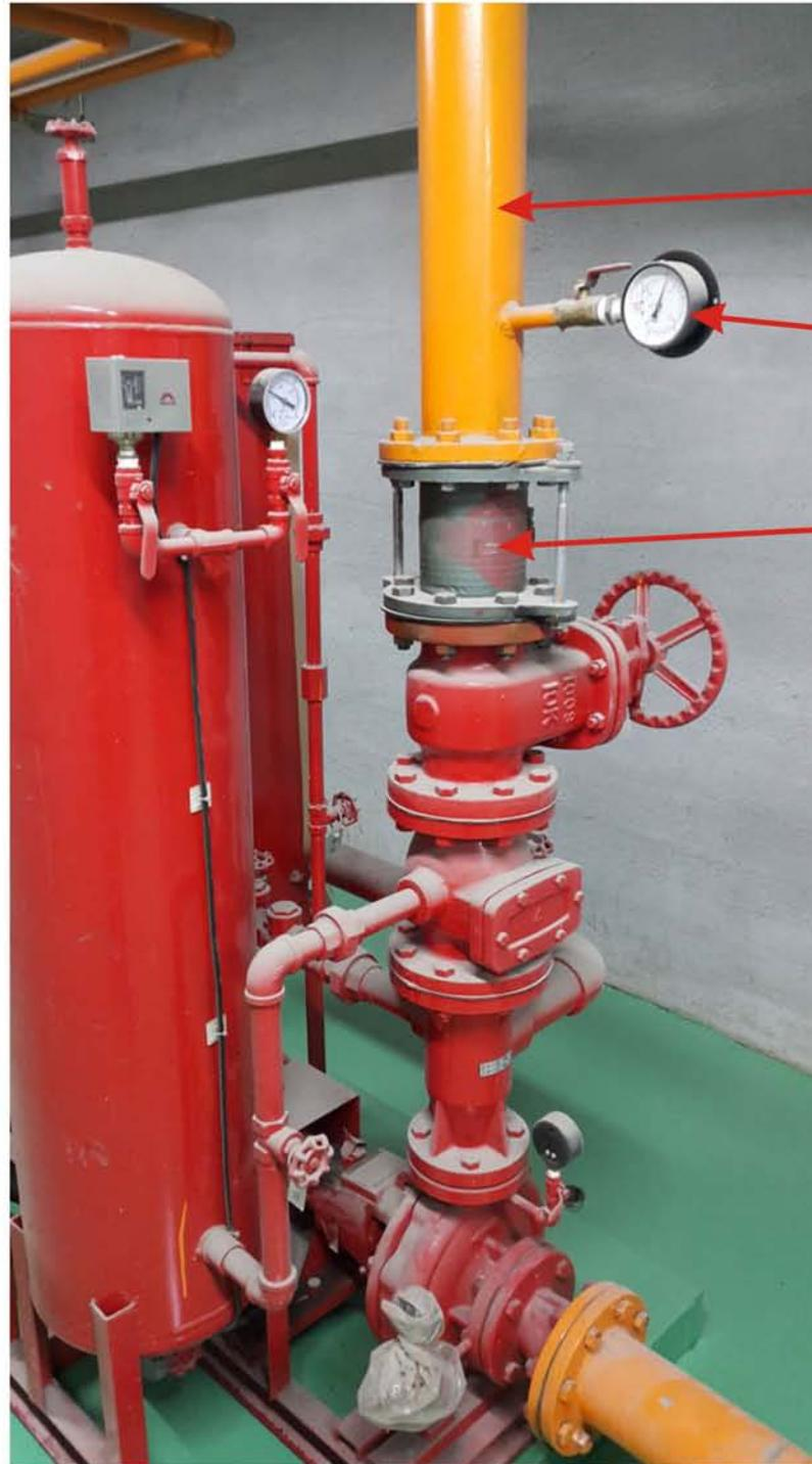
Connect **Main Piping** with SUS flexible joint.
