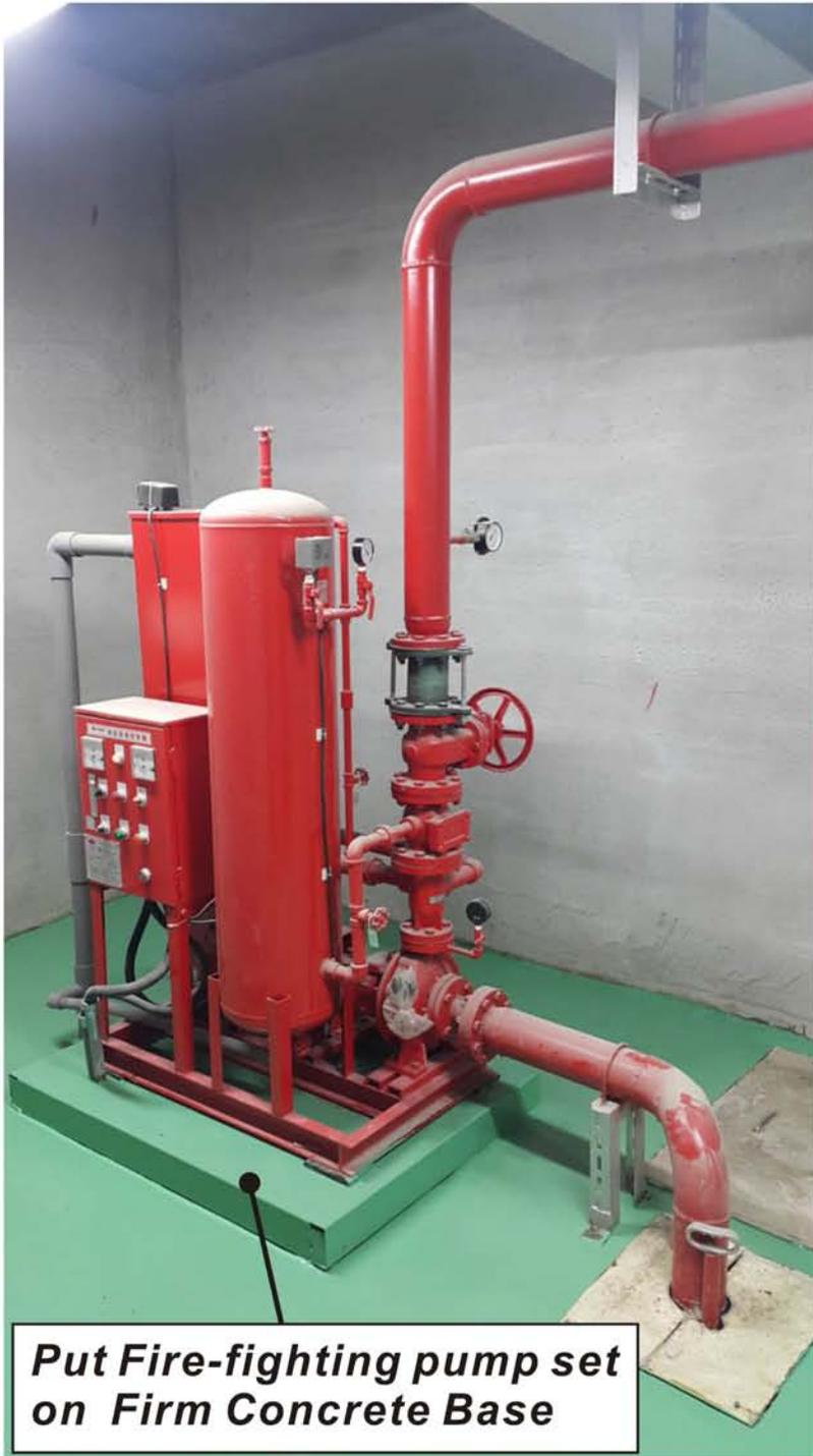
**Put Fire-fighting pump set on Firm Concrete Base**
